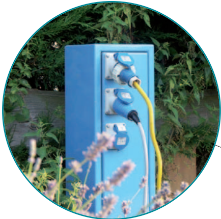
Plugging into the grid
