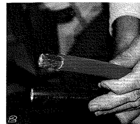
wiring was well under way. Begin work with batteries disconnected. Locating the position for the MasterShunt combined shunt and DC fuse (2) keeping the DC cables from
