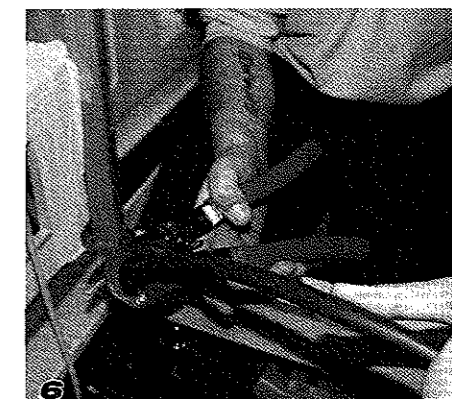
terminals are no longer recommended. With the MasterShunt in place connect the heavy duty cables for the shunt and fuse.
